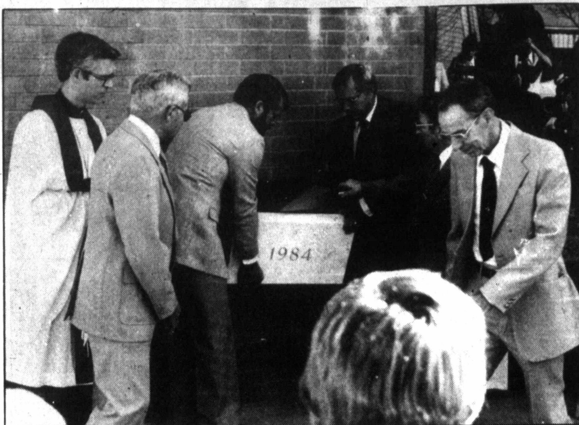
CORNERSTONE LAYING - The congregation of Zion Lutheran Church held a special service Sunday morning for the cornerstone laying in its new sanctuary addition currently under construction. Participating in the ceremonies are, center from left, Rev. Charles Paulson; Bruce Riehart, treasurer; Bill Hammer and Doug Beyer, placing the cornerstone in the building; Bob Lemke, building committee
