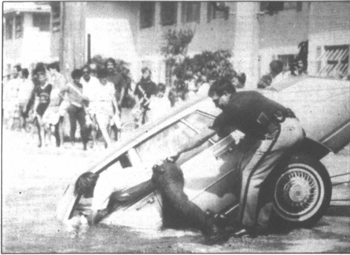
HELP!!! —The pavement at a busy intersection in Fort Lauderdale, Fla. bubbled and caved in recently when a water main broke, nearly swallowing a Cadillac but causing no injuries.
