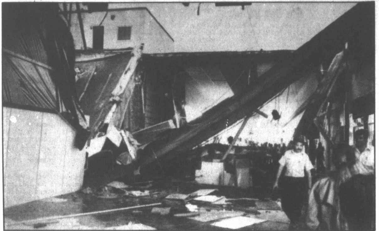
CAVE-IN—A roof of a theater caved in Tuesday in West Houston at the Memorial City Mall. Construction crews were in the process of renovating the theater to construct more stores
