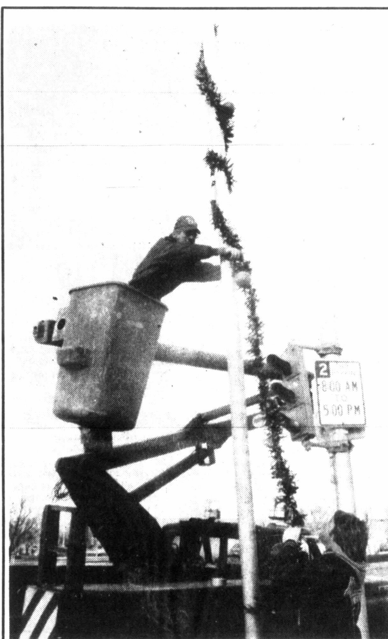
CHILLY WORK —Cold weather didn't stop installation of Christmas decorations in downtown Pampa Tuesday morning. City employees David Merica, on ground, and Melvin Chaney were busy putting up the holiday decorations despite the 25 degree temperatures. (Staff photo by Ed Copeland)
