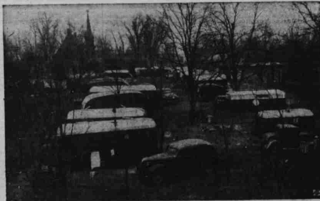
HOME'S WHERE THE TRAILER IS —Scarcity of living quarters coupled with the tremendous boom that construction of a new government powder factory has created makes trailer cities, like this one, an everyday sight in Charlestown, Ind. Charlestown's normal population is about 1,000; now 14,000 persons are building the factory, working on three eight-hour shifts.
