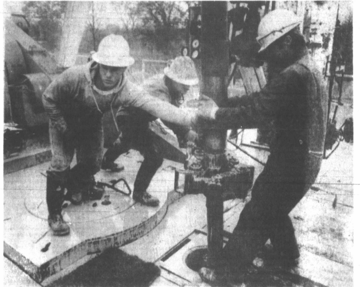
Roughnecks add another joint to a drill pipe in the Opelia Field near Athens. (AP Laserphoto)
