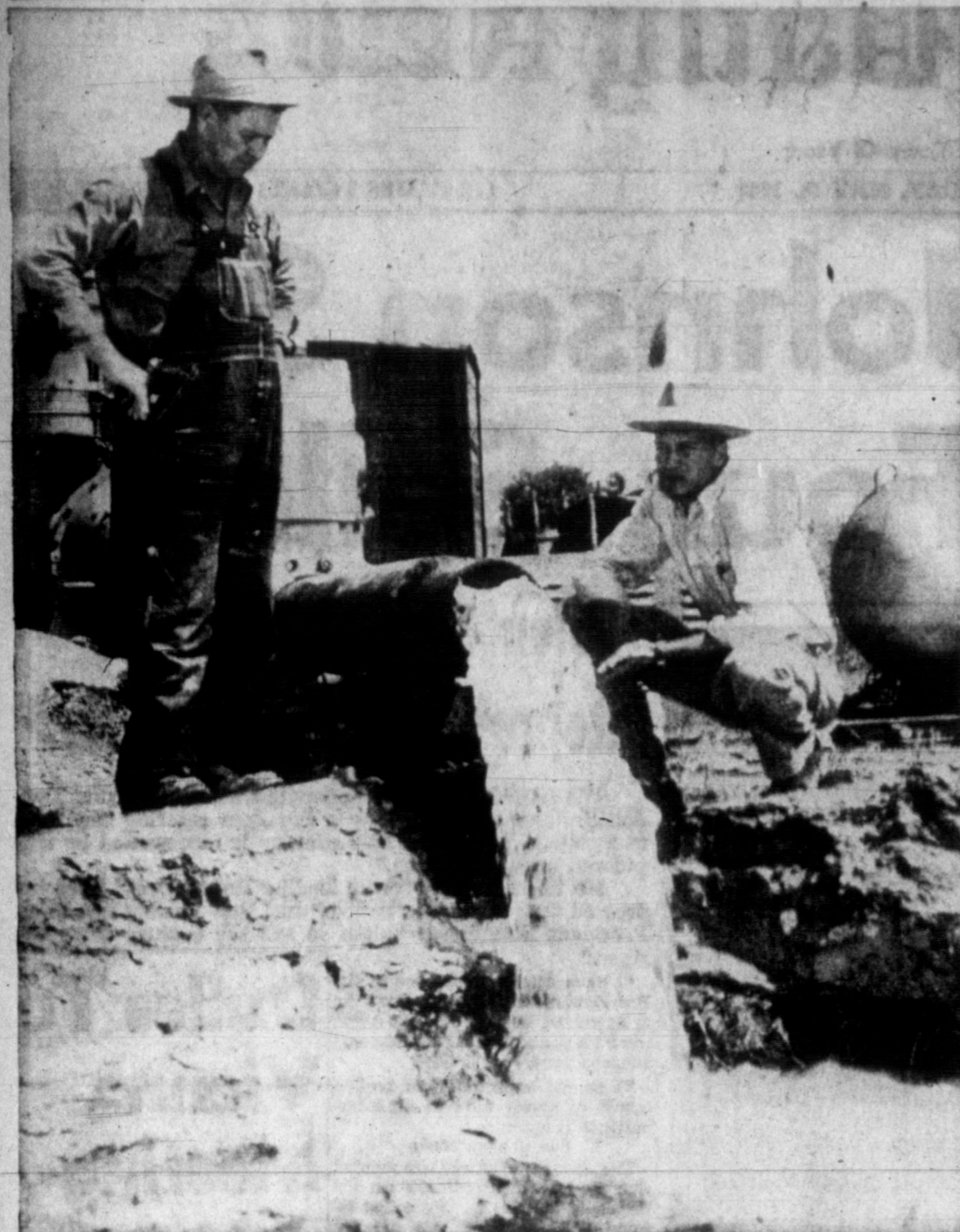
NEW WELL -- The new city water well for Lefors is currently running a 48-hour acceptance test and producing approximately 900 gallons a minute. The test is due to end today at 7 p.m. Looking on is city water superintendent R. L. Daugherty, left, and contractor Harold Courson of Kennemer - Courson drilling contractors of Pampa.
