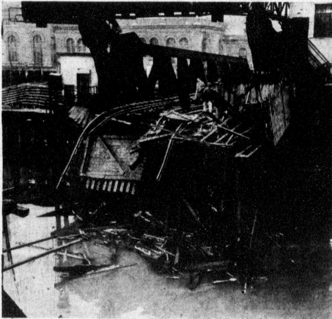
NARROW ESCAPE —Just after an oil tanker had cleared its span in the Chelsea section of Boston, a huge cement ballast block dropped from its mooring and crashed through the bridge. After creating this damage, the block sank in 30 feet of water.
