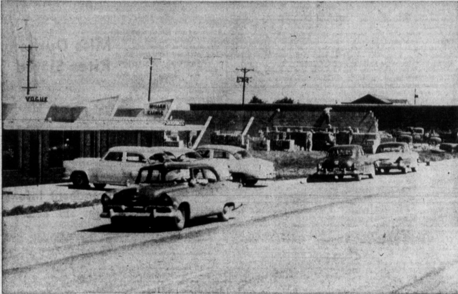
PAMPA BUILDS — Pampa is growing and good evidence of the fact is the construction on N. Hobart Street. Almost as far as the eye can see business establishments are going up. Several buildings under construction are the future homes of Vogue Cleaners, Bob Clements Cleaner's, Crossman Implement and Trail Electric. New businesses already in operation are Herlacher Construction Co., Koen's Portrait Studio, Highland Courts, Miller Chiropractic Clinic, Highland Pharmacy, Highland Children's Shop and the new Coca Cola plant. Other buildings are planned. (News Photo)
