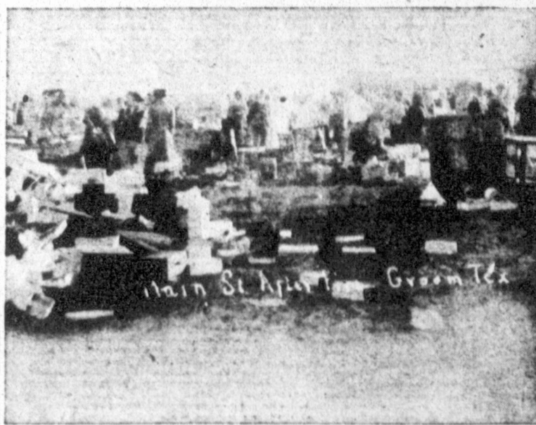
AFTER THE FIRE -- Goods and merchandise of all kinds are piled up in the middle of the street following the first big fire that nearly destroyed Groom. Modern fire fighting equipment is ready now to prevent such a disaster recurring.
