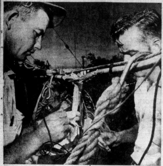
PHONES OUT? - Wayne Holt, cable splicer for Southwestern Bell Telephone Co., is working to get phones in the northwest part of town back in order. The cable was damaged recently by a power line and the moisture which fell in the night disrupted some phones. Holt's helper is Calvin McKinney. They are working 20 feet above the ground over West Kingsmill.
