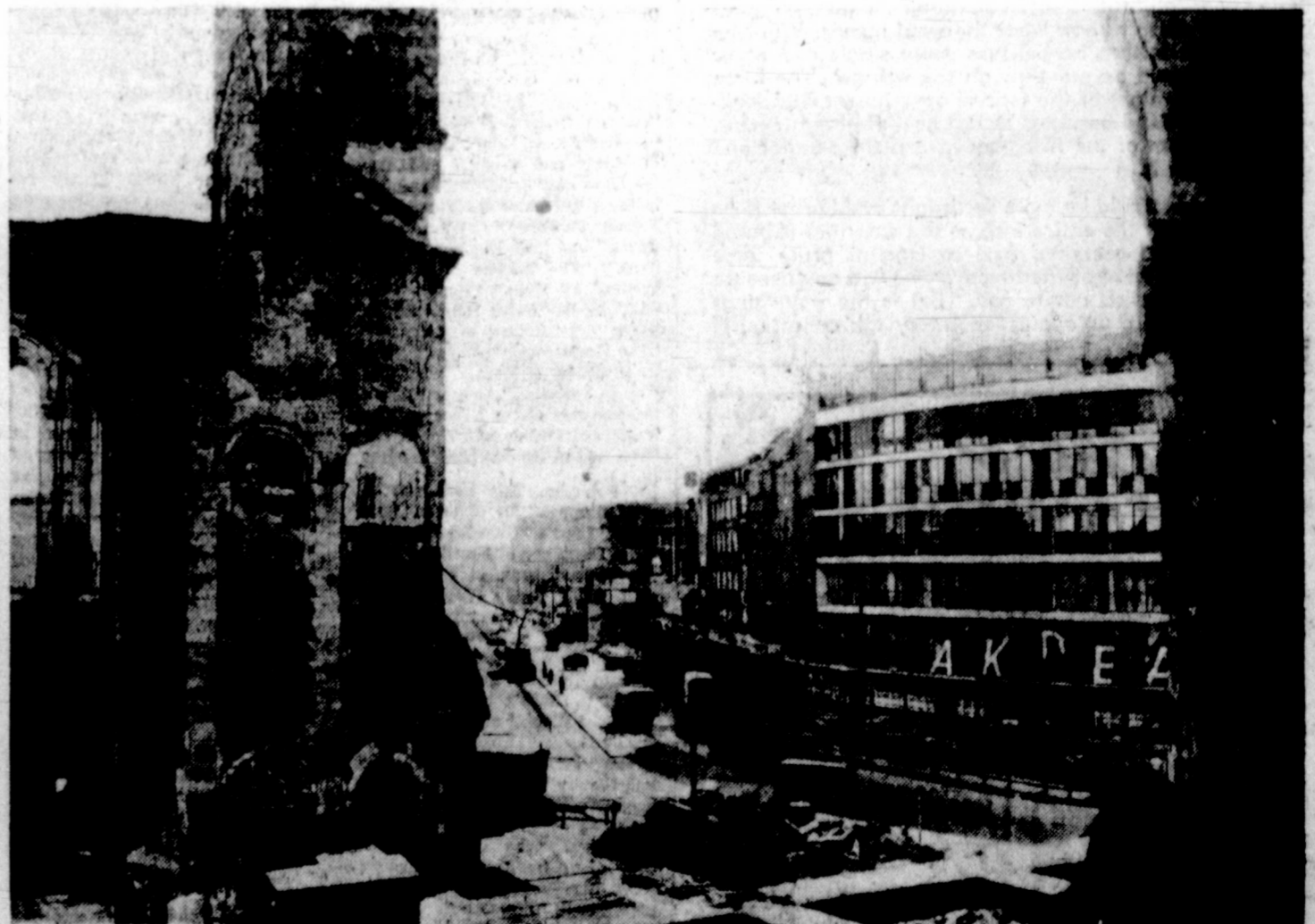
READY FOR BUSINESS —Reconstruction of war-torn Berlin is still in progress. Here, the lettering is being hoisted onto a new seven-story department store in the British sector, as seen from the ruins of Memorial Church. The wide thoroughfare, Rankestrasse, is the scene of considerable building activity these days.
