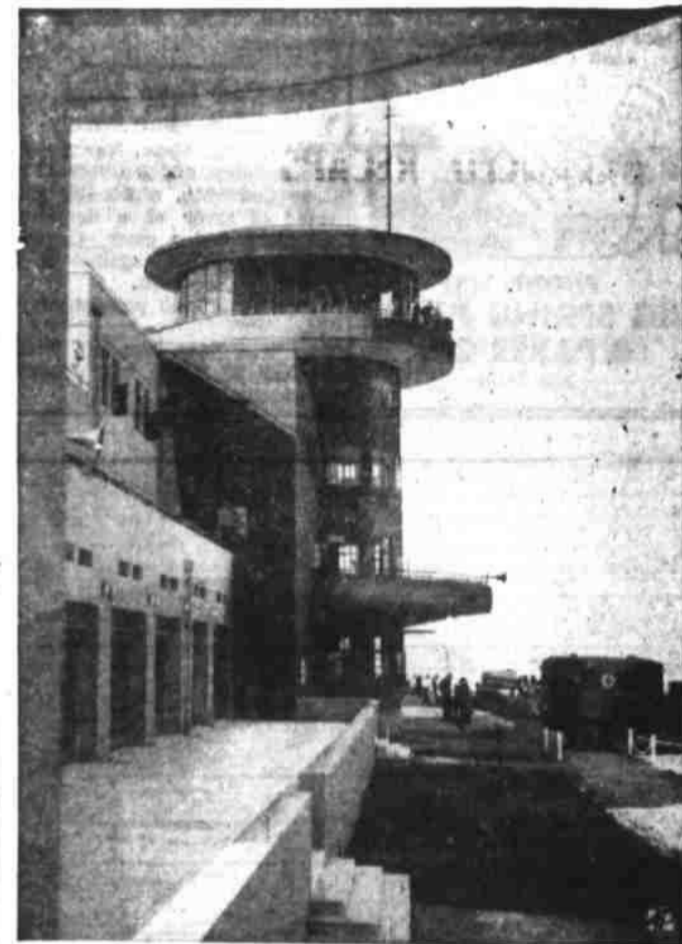
PALESTINE AIRPORT —View of the control tower of Lydda airport in Palestine, rated one of the most up-to-date airfields in that part of the world.
