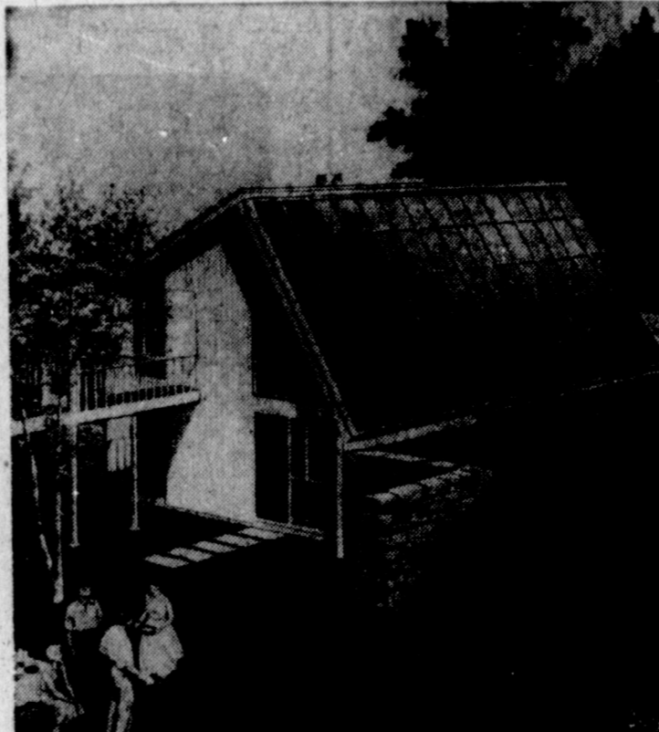
SOLAR HOUSE —Heat from the sun for an operating cost of about $50 annually has been achieved in the experimental house sketched above, a project of the Massachusetts Institute of Technology. Located in Lexington, Mass., heat collector beneath glass roof warms water of a closed system to about 150 degrees F. Water gives off heat through a heat exchanger, and can retain its warmth in storage for about three days. Heat exchanger operates to cool home in summer. Sketch is from Popular Mechanics magazine.
