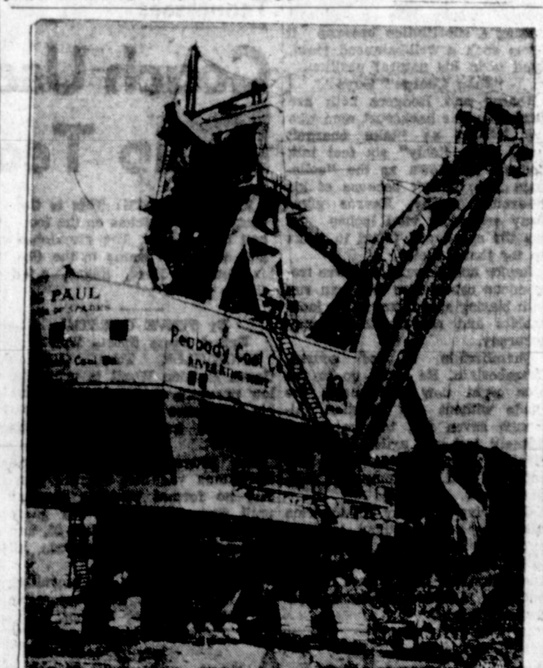
KING OF SPADES —"Big Paul, the King of Spades," is the first of three giant excavators to be put into operation by the Peabody Coal Company. Used in the company's new River King Mine near Freeburg, Ill., the stripping shovel can scoop up 105 tons with its big dipper, enough to fill two railroad cars.
