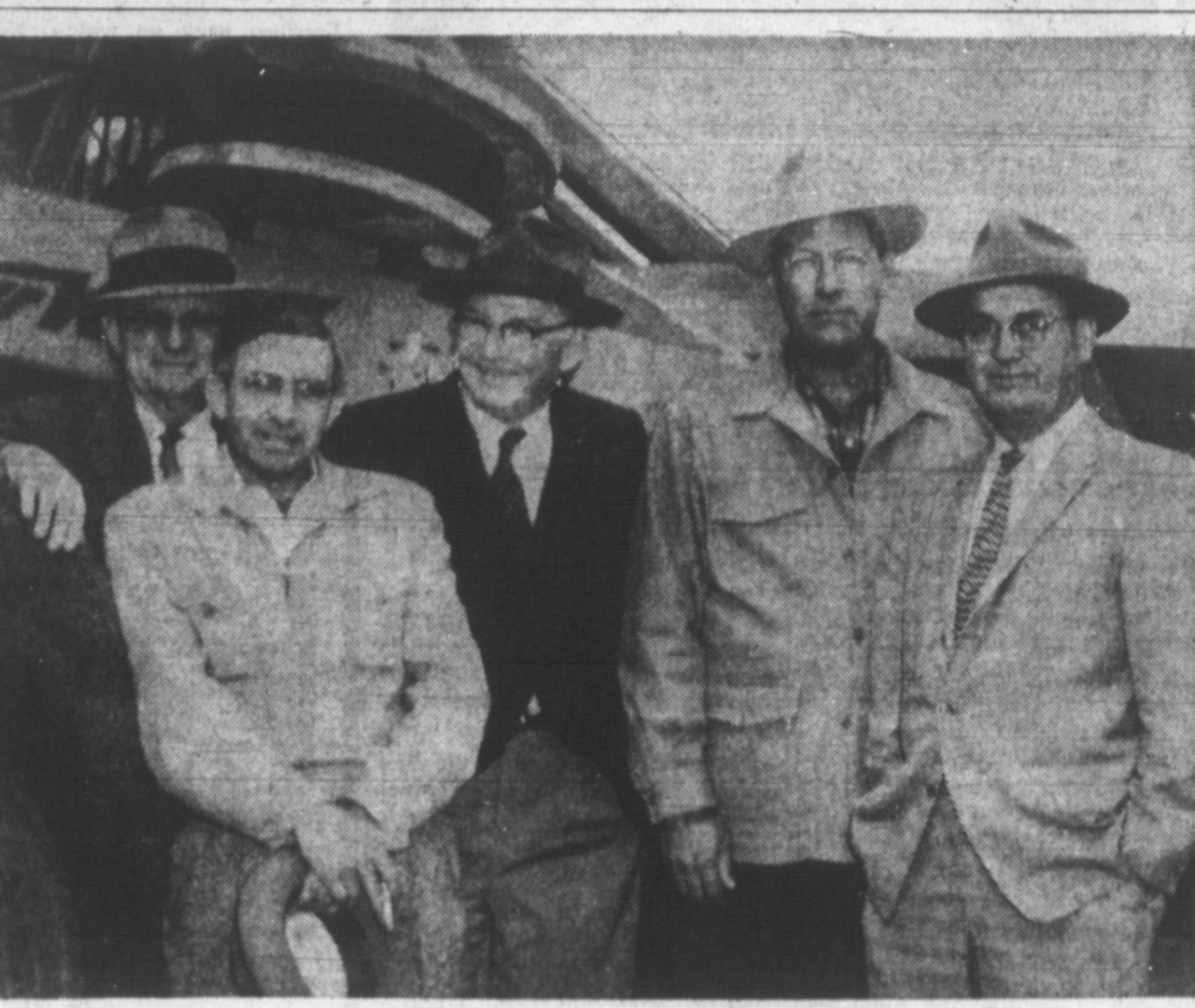
HOTEL GRADING WORK STARTS
