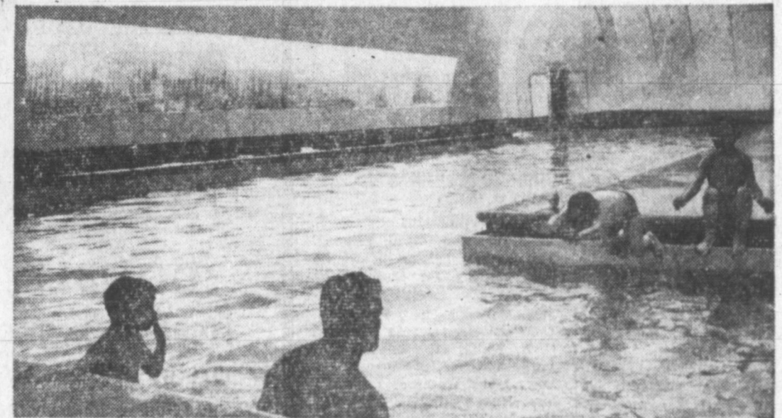
POOL PARADISE —A spot where swimmers can frolic all year, this indoor pool is located under a dome-like cover in Palo Alto, Calif. The cover is a vinyl-coated, nylon convertible affair that's easily inflated. It's anchored at the base by a water-filled tube.
