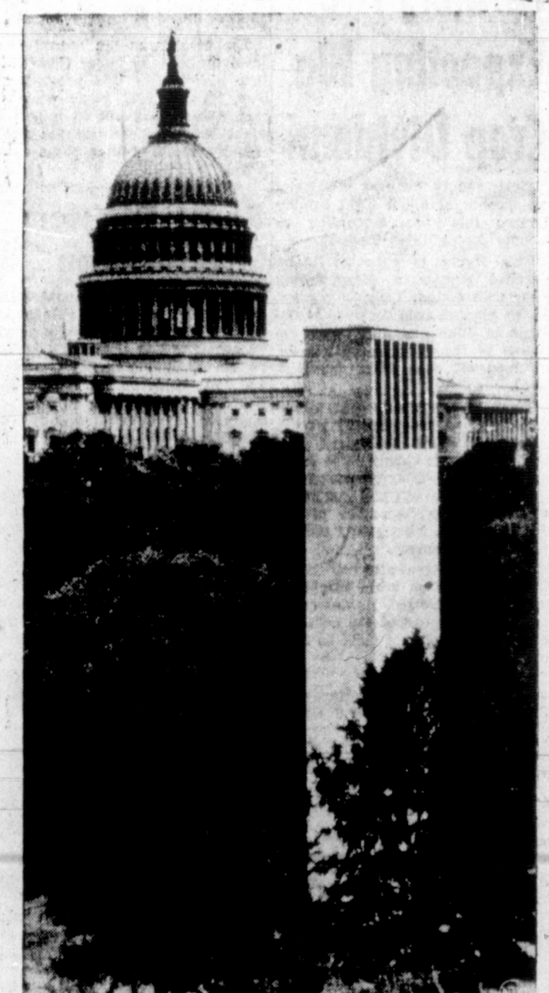
A NEW LANDMARK —Against the background of the Capitol stands the Robert A. Taft Memorial tower, latest monument to be erected on the Washington scene. The structure is 100 feet high and contains a 27-bell carillon. It was constructed at a cost of over $850,000, obtained through private donations.
