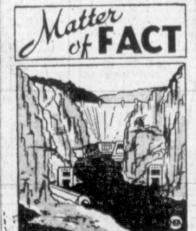
The world's highest dam is the Mauvoisin, on the Dranse River in Switzerland. It was completed in the fall of 1957. The dam is an arch type, of concrete, 780 feet high. The dam was built to supply power. Hoover Dam, on the Colorado River, between Arizona and Nevada, at 726 feet, is the second highest water barrier. O Encyclopedia Britannica
