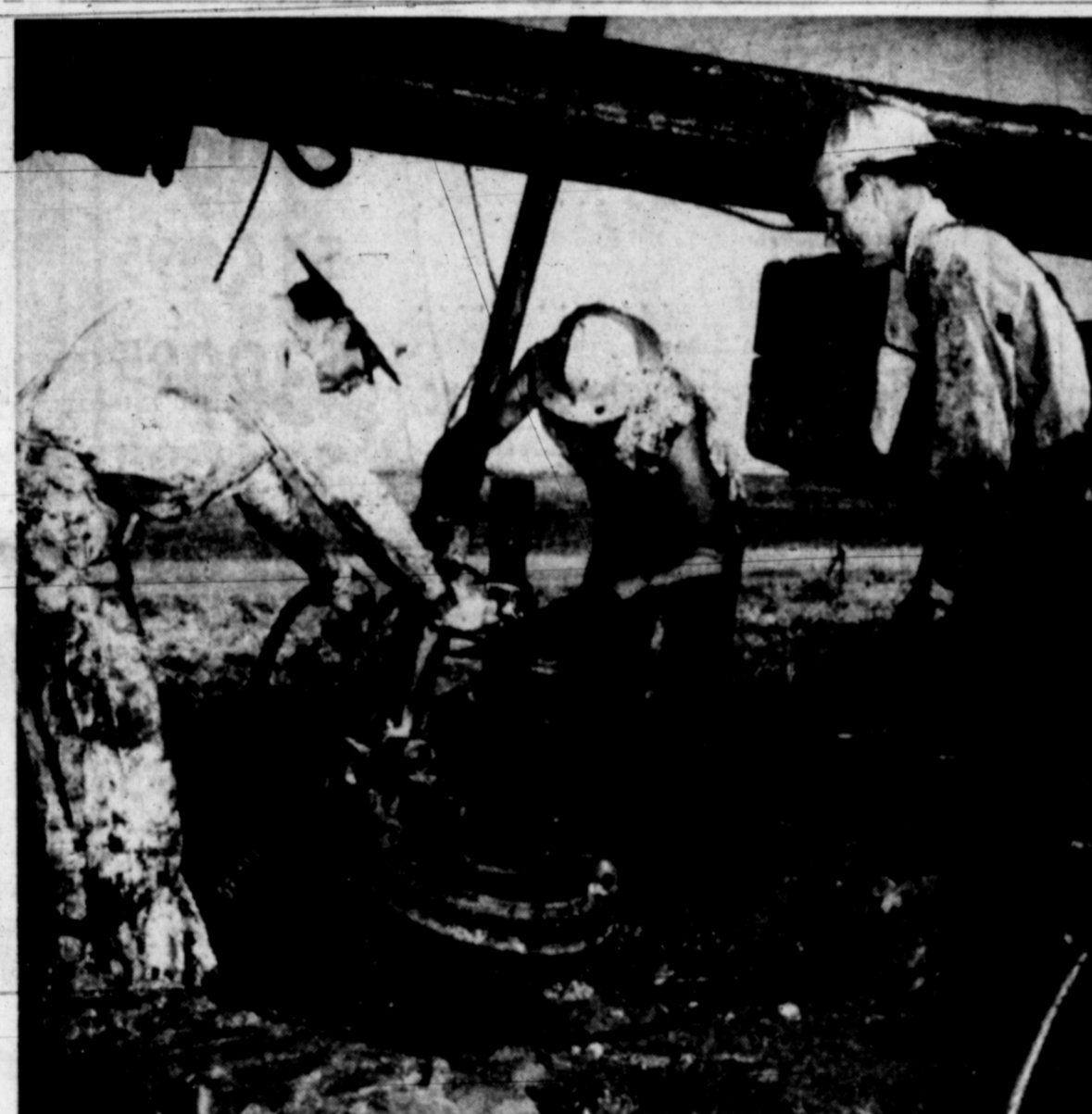
CLEANING UP THE DEBRIS
