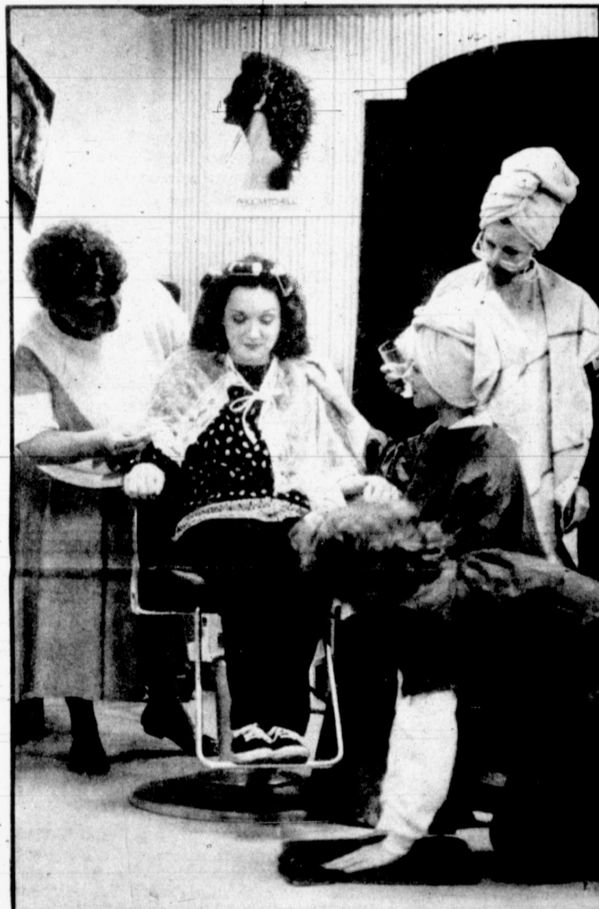
Everyone goes to work when Shelby (Kelly Yeary), seated in chair, lapses into insulin shock while having her hair done on her wedding day. Pictured from left are, Truvy (Sandy Crosswhite), Shelby, M'Lynn (Dee Dee Laramore), Clairee (Marquette Wampler), and Annelle (Sheila Luther) who is wiping spilled juice from the floor.
