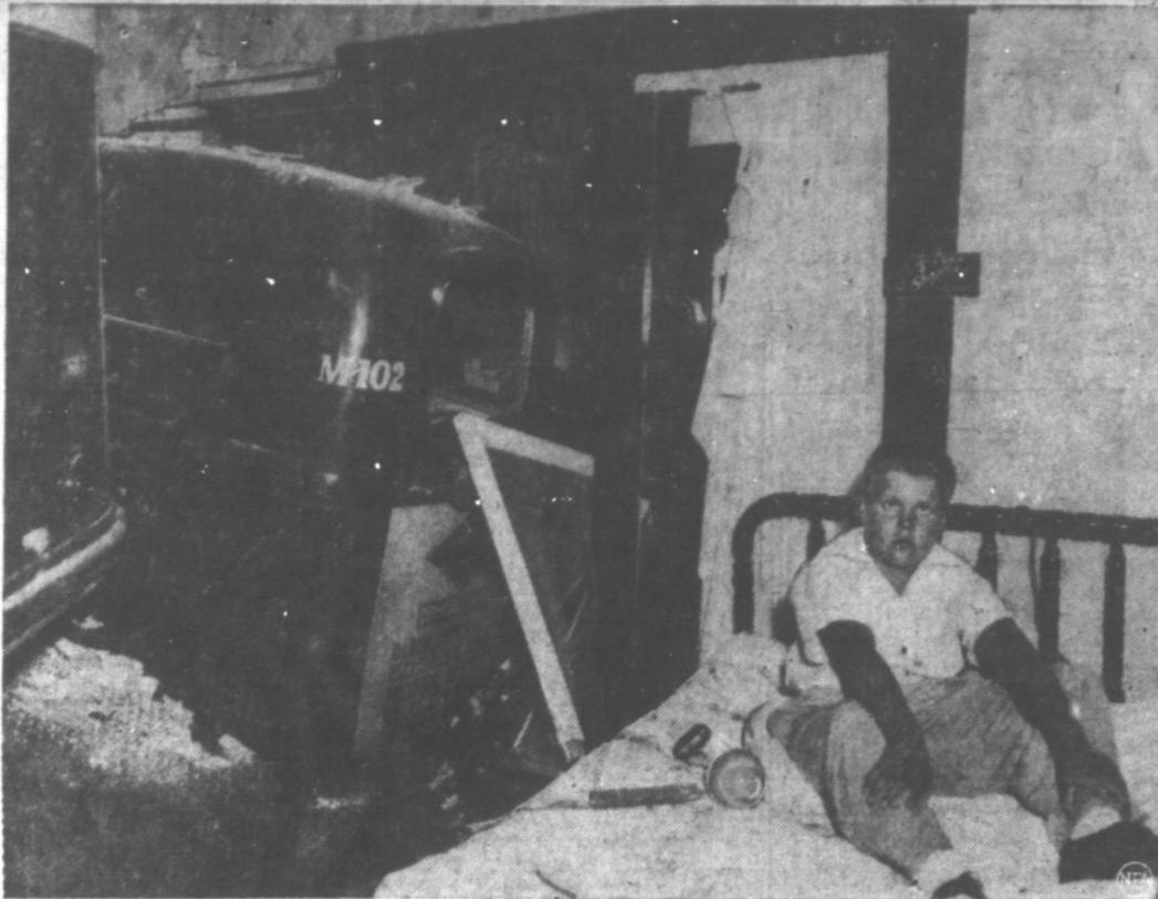
Billy Bruns, 11, sits on the bed in which he was sleeping when a 17-ton trailer truck skidded off the highway in New Bremen, O., and crashed into his bedroom. The truck ploughed into the house, just missed Billy, and slammed into the dining room beyond. Note the sign over Billy's bed: "The Lord is my shepherd." The driver, Lester Snodgrass of Chicago, escaped with scratches.
