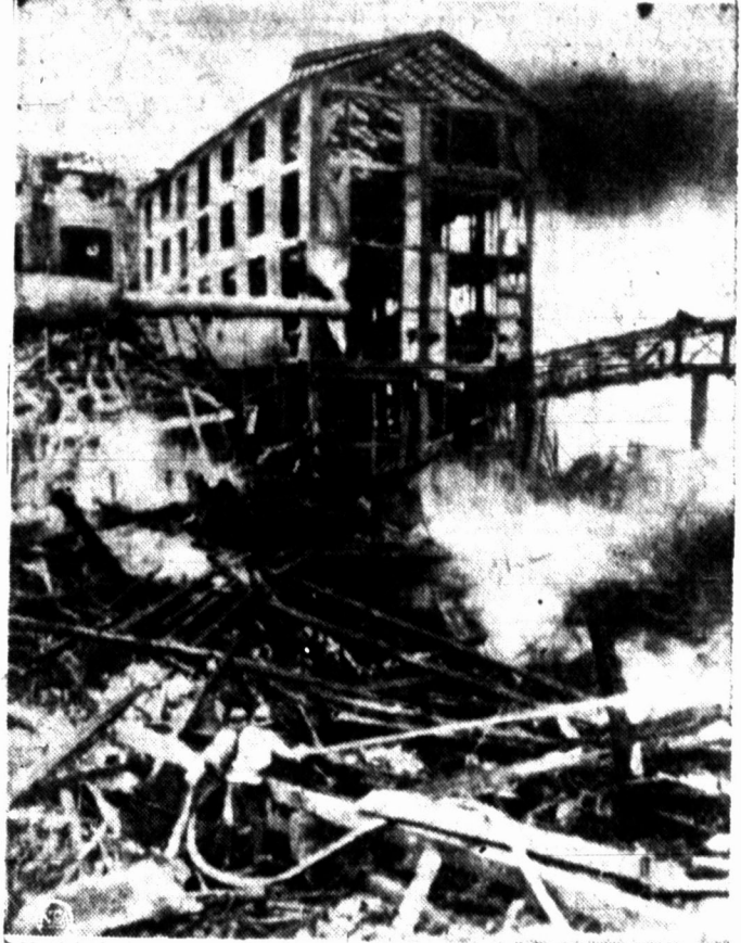
FIGHT FIRE IN FARBEN RUINS—Firemen, lower left, pour water on the burning ruins of the I. G. Farben chemical works at Ludwigshafen, Germany, which exploded as workers were preparing to go off work for the day. American, German and French rescue workers raced to the scene to search the wreckage for injured and dead.
