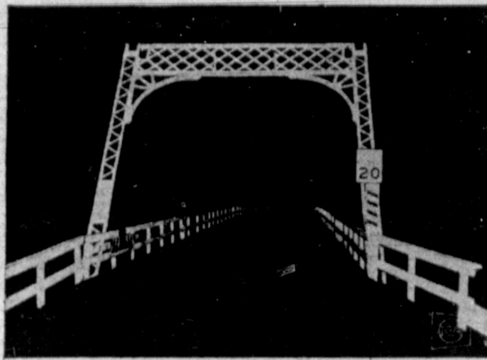
tricked up a bridge near Minneapolis, Minn., to make it safer. At left, as it looks in the daytime. At right, its appearance at night. A reflective liquid applied on the structure glows brightly when the lights of an oncoming car strike it.
