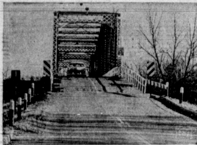
IT'S AS PLAIN AS DAY — Bridge approaches are danger points on rural roads. In many cases, the highways zoom quickly to new levels and driving areas narrow to accommodate the outdated spans. Chalk up some progress in attacking this problem. Engineers have
