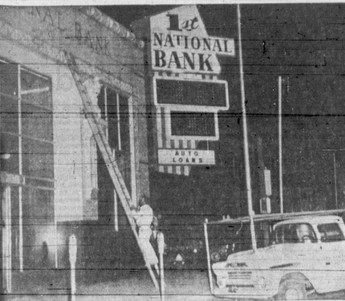
TIME AND TEMP — Workmen Friday night installed the new First National Bank sign at the corner of Cuyler and Foster sts. The 1800-pound sign was delivered Wednesday...
