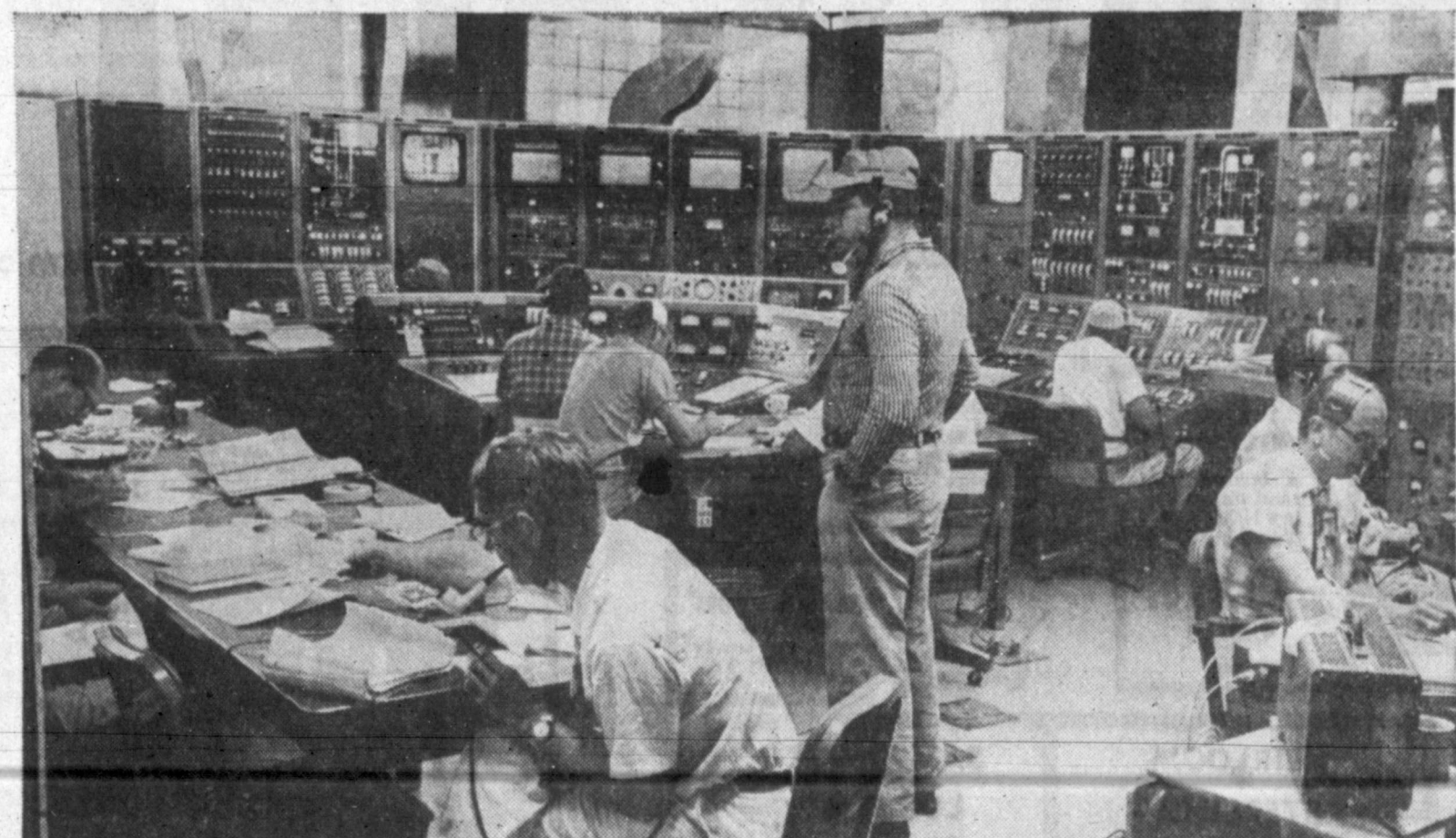
Control room at Nevada Test Site for conducting nuclear rocket propulsion experiments operates under the direction of the Los Alamos Scientific Laboratory. During reactor power runs, nearly 600 signals are fed into the room from
