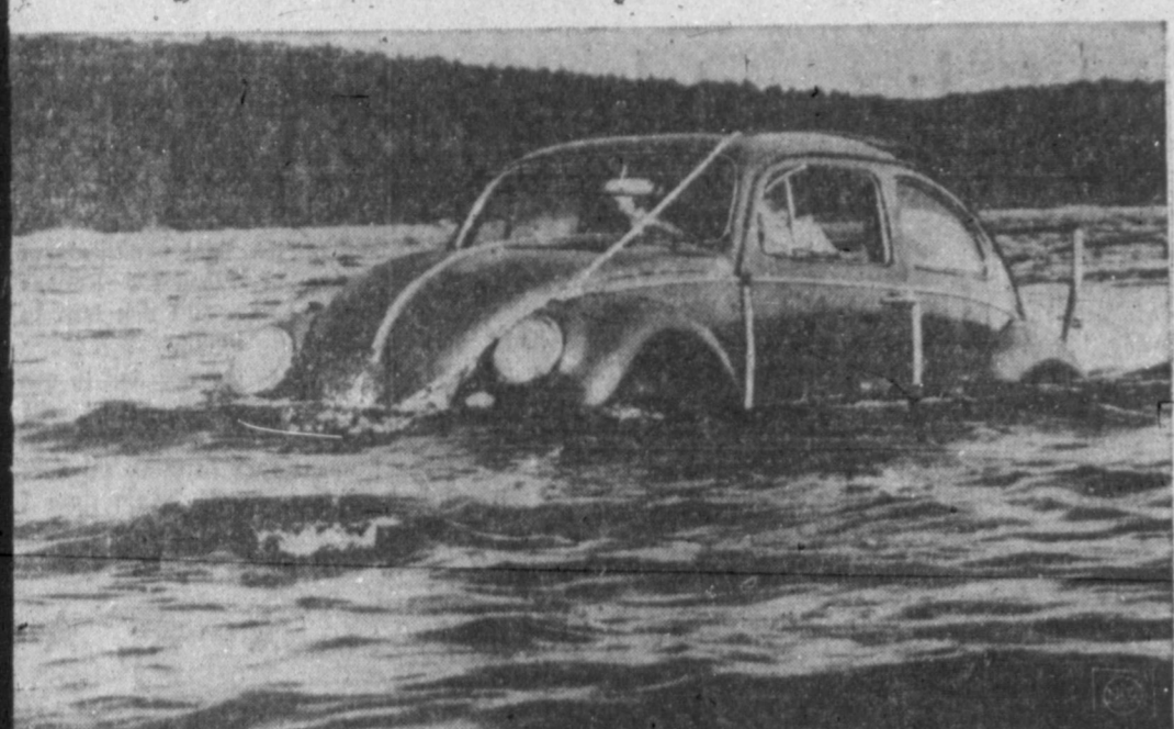
FLUID DRIVE—Volkswagen putt-putts through Lake Malar in Sodertalje, Sweden. The auto was turned into an amphibian by making the body watertight, extending the exhaust and air inlet pipes above the waterline and adding a propeller.
