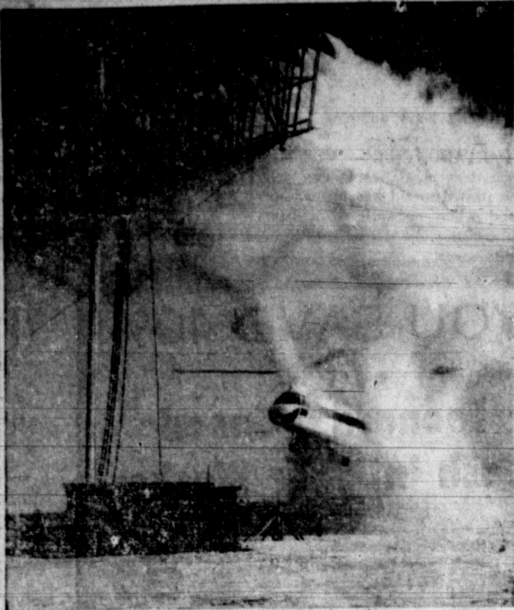
COLD SHOWER —Chilling water vapor engulfs a Boeing Vertol 107 as the helicopter undergoes a rigorous de-icing test at Canada's National Research Council near Ottawa. A spray-rig on the left produces a vapor cloud, which sub-freezing Canadian weather quickly condenses to ice on the helicopter's rotor blades. An electrical de-icing system is then activated. Heated strips running along the blades' leading edges cause the ice to loosen and the whirling motion of the rotor blades sheds the thawing ice.
