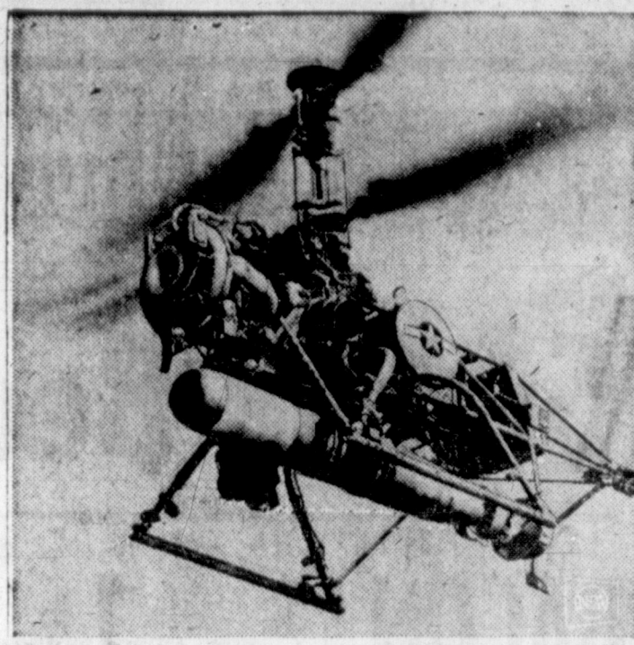
DRONE WITH A STING —A drone helicopter on sea operations test off Long Beach, Calif., carries the Navy's new solid rocket fuel torpedo MK 46-0 under it. This type antisubmarine torpedo can be launched from a helicopter, fixed wing aircraft or surface craft.
