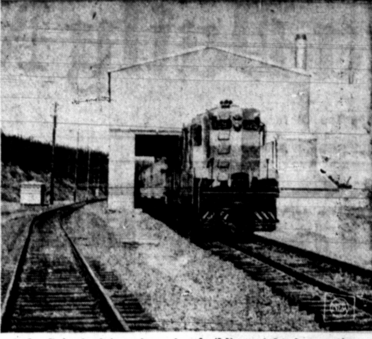
is loaded. Arriving at crusher building, right, locomotive precisely spots and dumps each car in turn—automatically, without human intervention. Starting, stopping, speeds and routes, dumping—even bell ringing—are all dictated by an electronic brain.
