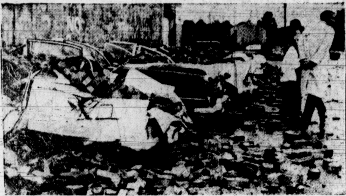
WIND DAMAGE — A 98-mile-per-hour wind roared through Fort Worth, Tex., over the weekend and left in its wake damage estimated at $1.5 million. Seven persons were hospitalized. At the Hereford Hotel, on the north side of the city, six cars were crushed by brick when part of the west wall collapsed in the high wind. The general adjustment bureau said today insured losses from Sunday's tornadoic winds and hail would exceed $500,000 but would probably be less than $1 million. No estimate of uninsured losses was made. Earlier reports indicated winds caused damage ranging upward to $2 million. The bureau is a non-profit insurance adjustment agency. W. J. Mahoney, manager, estimated 600 to 700 buildings were damaged by the storm. City officials estimated it would take a week to clean up the storm's debris. (NEA Telephoto)
