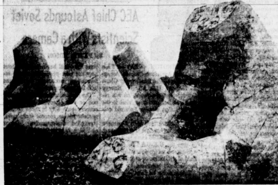
TONS OF FUN —Nigel Sayers, 3 peers out from an odd looking piece of concrete at Shoreham-on-Sea, England. Called stabs, they interlock and are used to form a slope to guard the beachfront against the battering sea. Nigel appears to think that they make fine playthings, even if they do weigh seven tons each.
