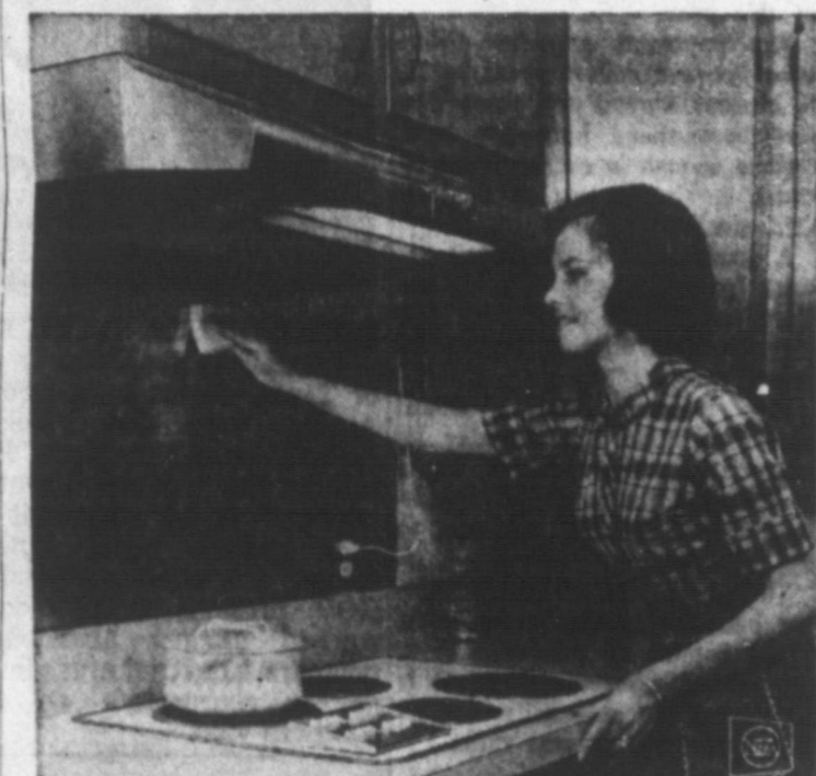
Boon to cleaner kitchens are range hoods. This no-duct hood filters cooking steam and odors through aluminum mesh and charcoal. Splash plate matches hood top.
