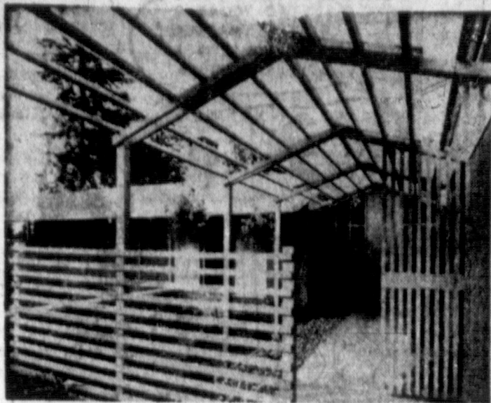
Artistically designed front walk makes entering this home a pleasant adventure. Walk is emphasized by canopy of slender Douglas fir posts and beams topped with rain cover of plastic panels. At front, near street, airy screens of spaced 2x2s give sense of enclosure to exterior entrance way. Beds of river rock and greens border walk.
