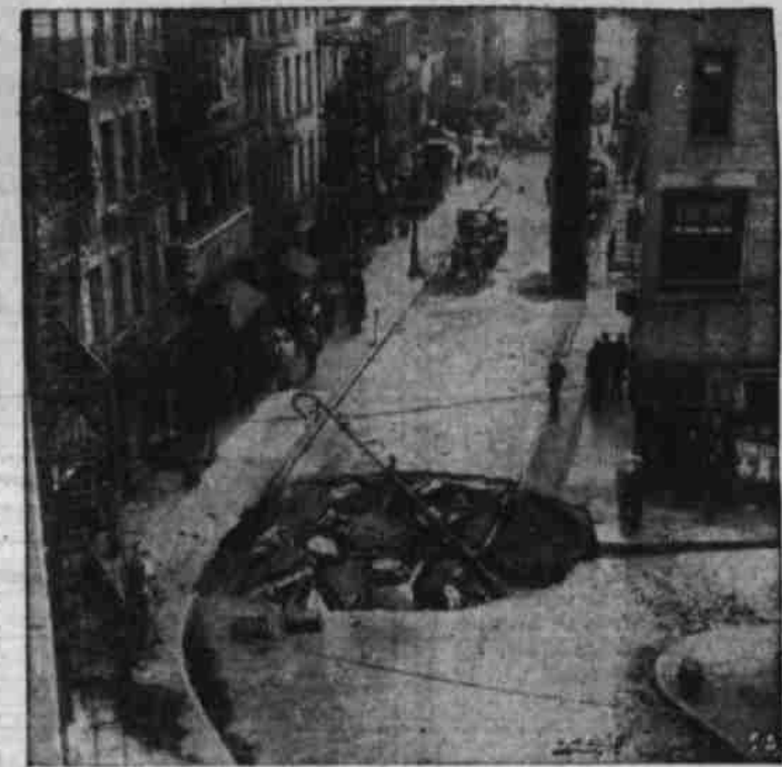
NO, NOT A BOMB —A water main break and gas explosion, not enemy action, made this hole in the paving at Mott and Pell streets, in the heart of New York's Chinatown.
