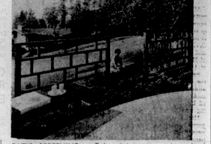
PATIO SCREENING -- Only minimum screening is needed for privacy when patio is above grade and above direct sight line from neighboring homes. A pair of offset western red cedar screens in an open pattern does the job here. Shrubbery will fill in at the base for additional screening action.
