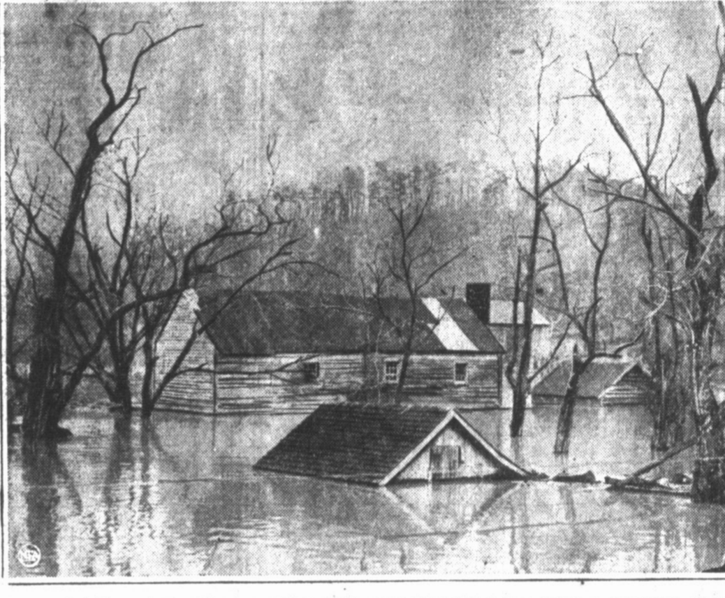
The beautiful Shenandoah valley was hard hit by flood waters that swept over a dozen states, took more than 50 lives and did untold damage. Sights like that pictured above near Winchester, Va., with farm buildings inundated to the roof, were common along the banks of the Shenandoah.
