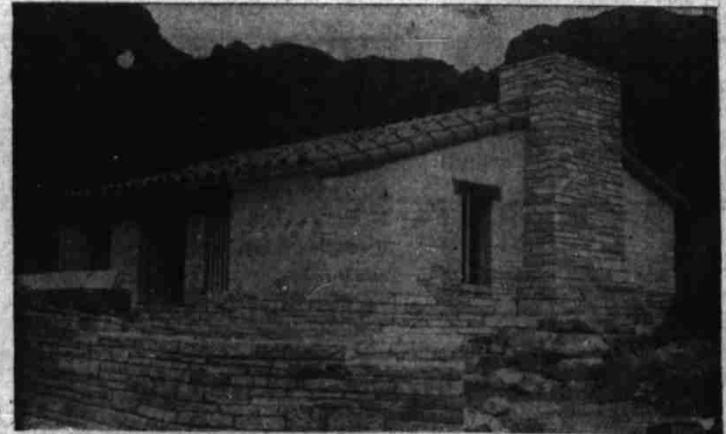
READY FOR TOURISTS SOON—This is one of the luxurious cabins being built in the Big Bend National Park by CCC workers. This and another cabin are practically complete and work is being rushed on several others.
