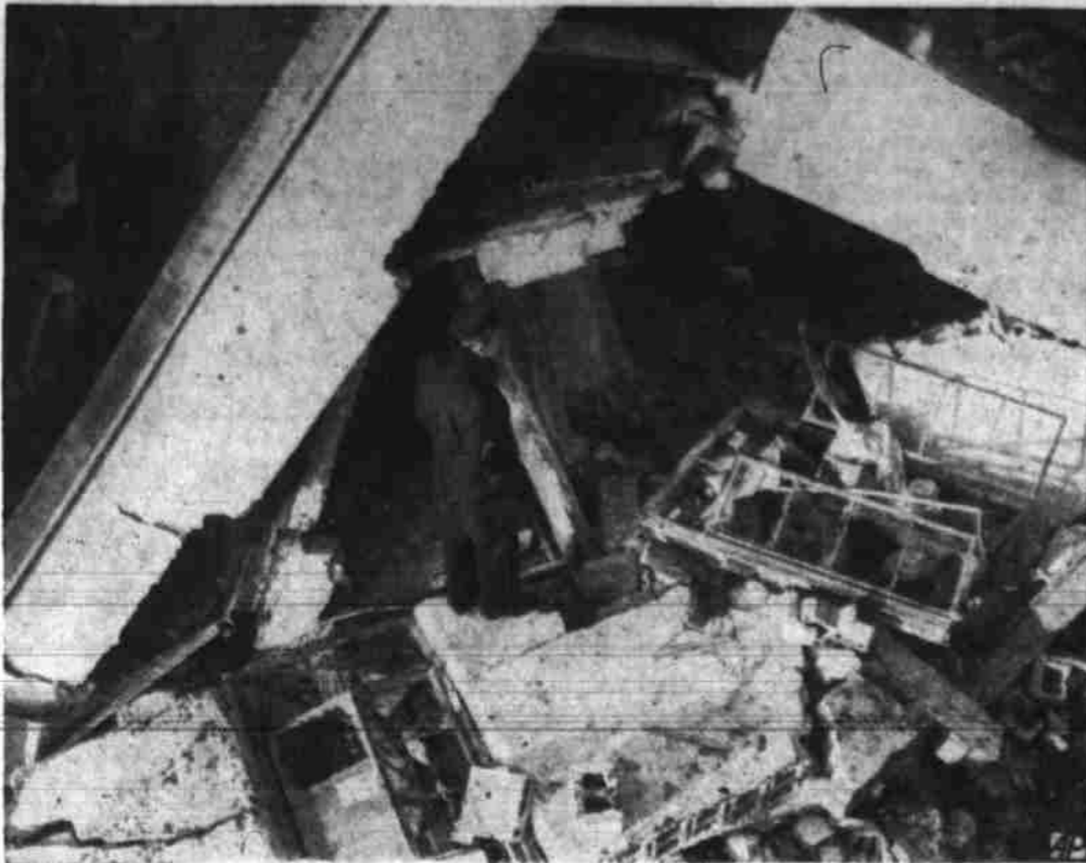
APARTMENT HOUSE BLAST INJURED 14—A policeman looks at the wreckage of the four-unit apartment house in Dallas, Tex., which was wrecked by a blast of undetermined origin. Fourteen persons were injured. The walls were blown outward and the roof collapsed to make an inverted V. (AP Photo)
