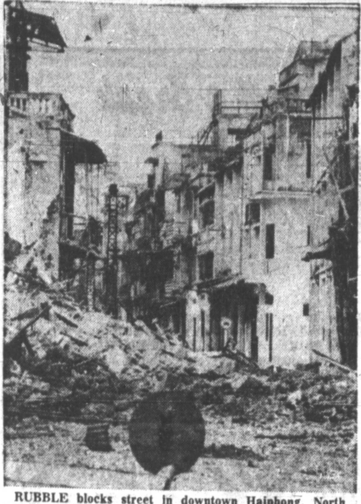
RUBBLE blocks street in downtown Haiphong, North Vietnam, after U.S. air raids. Photo released by Japanese news agency shows bomb sign in foreground, indicating there are unexploded bombs in area and that it is "off limits."
