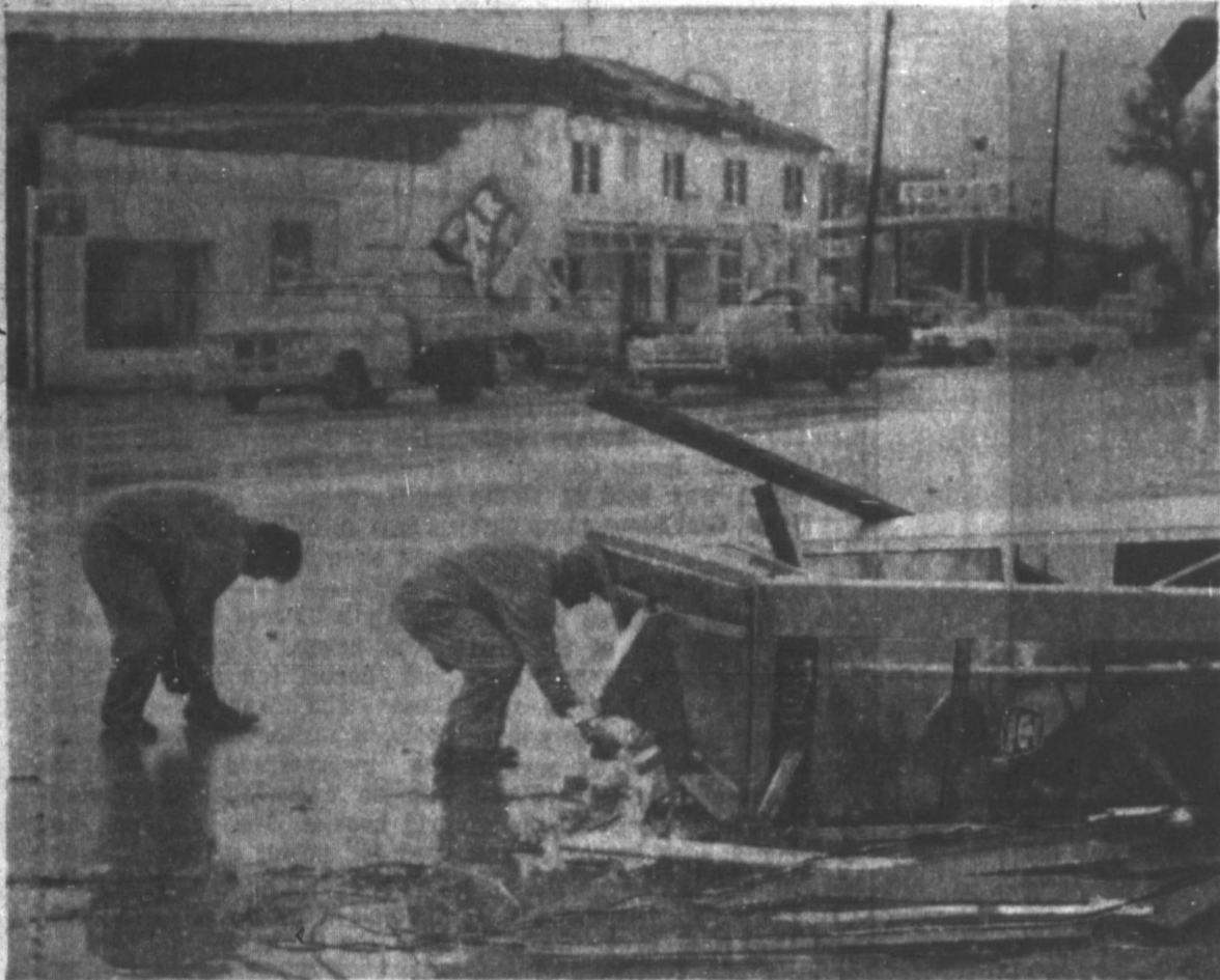
STORM DAMAGE — Workmen are shown here cleaning up after yesterday's tornado at Miami. The telephone booth in the foreground lies partially in the main street of the town and the damaged hotel is shown in the background.
