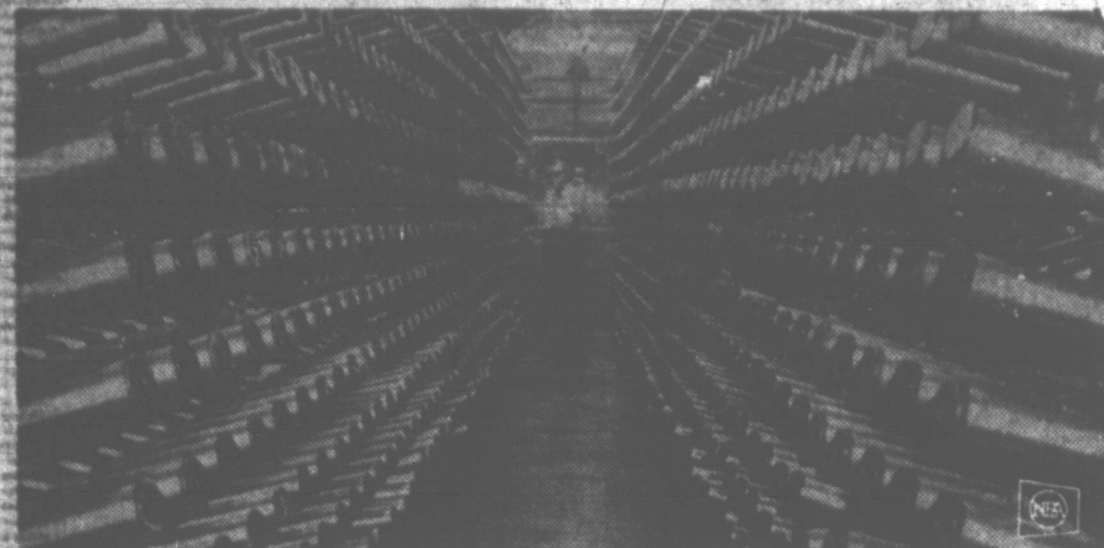
SPOOLS OF TIRE CORD feed a power loom weaving tires at the textile mill of the Goodyear plant in Cedartown, Ga. The tire industry in the United States is expected to consume about 500 million pounds of polyester, rayon and nylon fabric this year.
