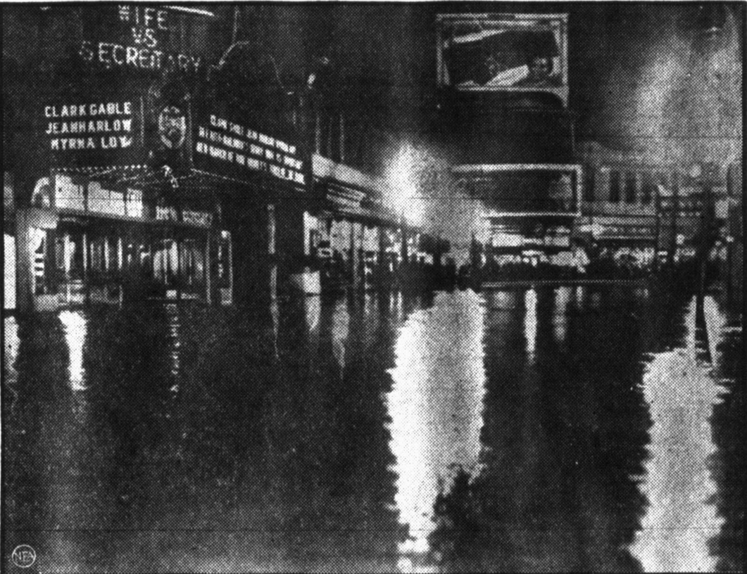
Water poured into this deluxe movie theater in Pittsburgh's downtown area as the flood rose to a depth of 18 feet in some places in the famous "Golden Triangle." Damage in the beautifully-decorated theaters and stores, was especially heavy. Windows crashed in before the mighty impact of the surging waters. Occasional rowboats passed up and down the lagoons which had been busy streets a few hours before.
