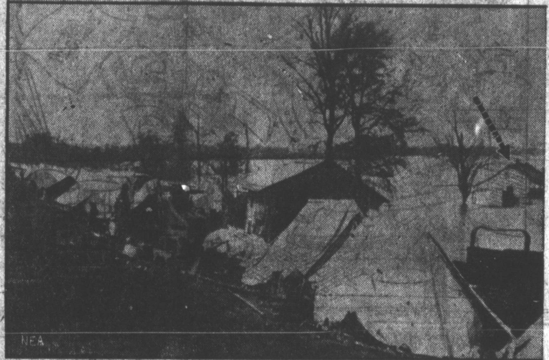
Here is the first picture of the widespread destruction and suffering caused by a break in the Mississippi levee near Laconia, Ark. Large areas inundated by the flood waters and thousands were driven from their homes. This picture shows a refugee camp near Laconia, tents being used as temporary homes. The flood waters are even menacing this camp. At the extreme right an arrow points to a house with the water up to the roof.
