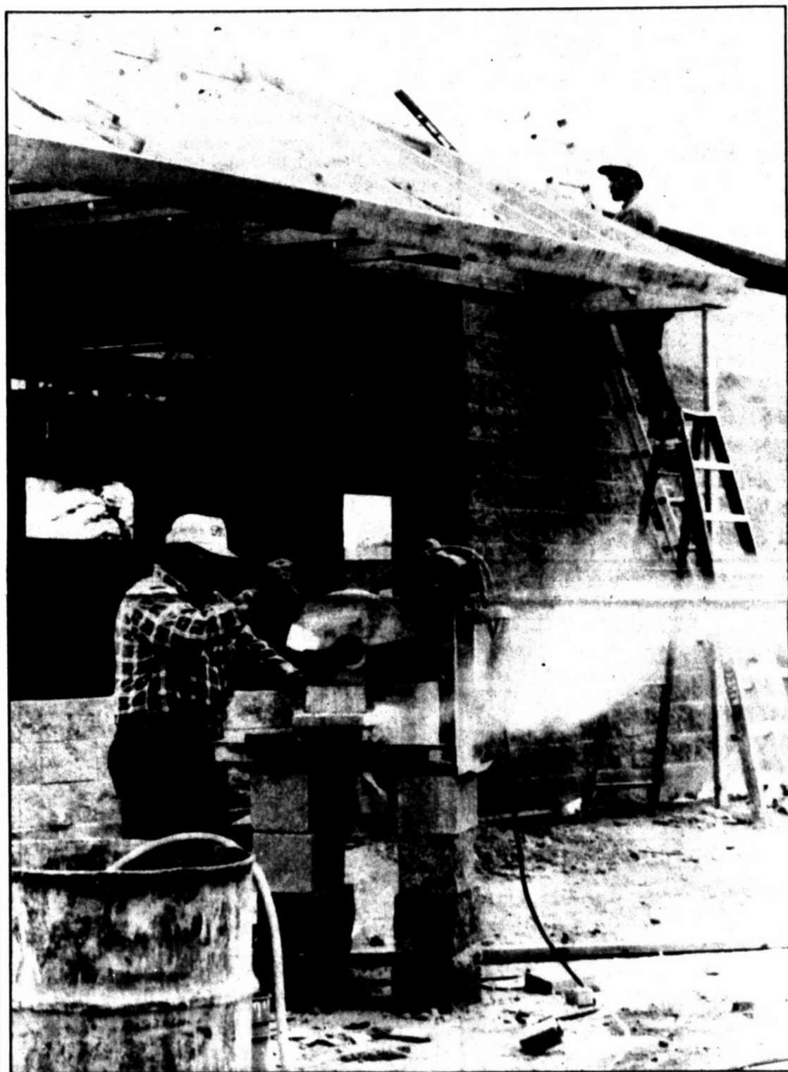
Victor Diaz with Carl and Charles Buccola Masonry uses an electric saw to cut a cinder block for placement on the new McDonald's restaurant under construction at Somerville and Hobart. Under construction by Kelly Wood Co. of Amarillo, the fast-food restaurant, replacing the former one which was severely damaged by fire this past winter, is due to open next month. (Pampa News photo by Darlene Holmes)
