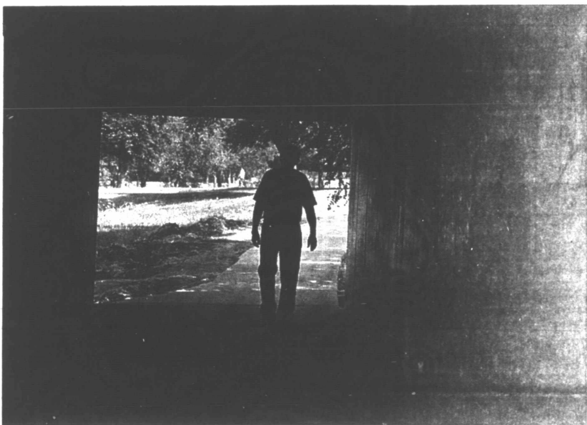
Reed Kirkpatrick, director of Pampa's Parks Department, is silhouetted in the newest update of the city's hiking and biking trail system. The tunnel Kirkpatrick is walking through, inspecting the newly poured concrete walkway, is in Central Park beneath Louisiana Street.
