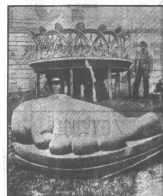
Before being shipped to America (as a gift from the French people) Liberty was set up in Paris and sightseers permitted to clamber up to the torch. The immense size of the Statue of Liberty becomes apparent through comparison of the man with the ornamental work for the torch and the huge toe sections. The Statue of Liberty came into existence piece-meal in the studio of sculptor Bartholdi in Paris, where an old sketch shows the work on hand and torch in progress. A rare closeup of Liberty's head is provided in this picture, made before the statue was completed. Set up in the French capital, it dwarfs the men standing on the pedestal.
