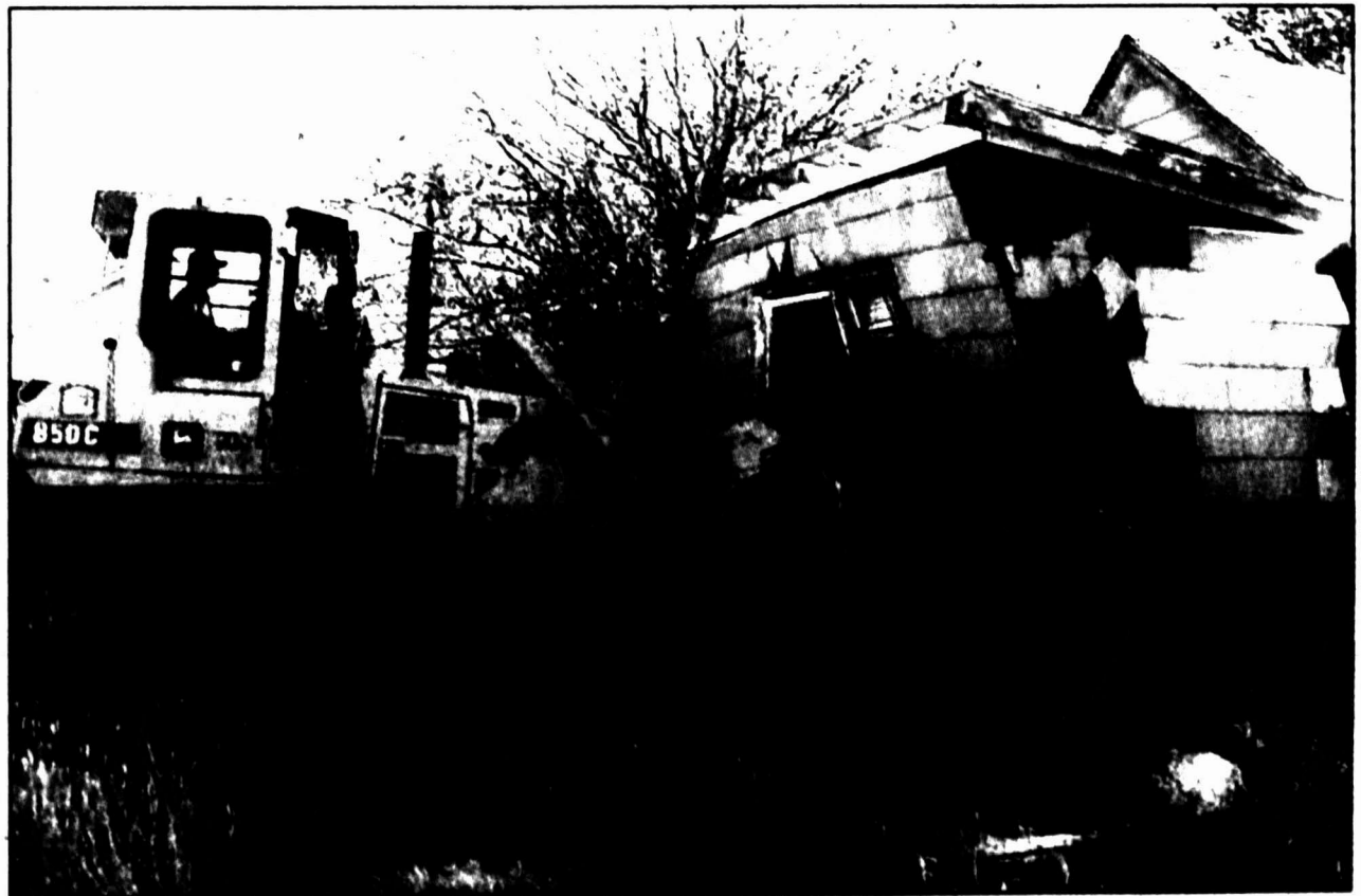
Israel Ulloa of the Pampa Street Department tears down another junked house, this time on Browning.
