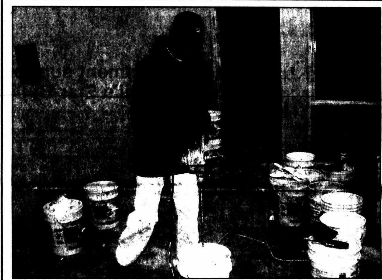
Robert Abernathy is mixing wallpaper paste getting ready to paper walls in the new Clarendon College Pampa Center on West Kentucky. The building is scheduled to be open and have classes in January.
