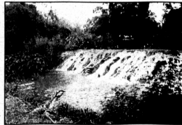
18th Century dam built to divert the flow from the San Antonio River to mission Espada.
