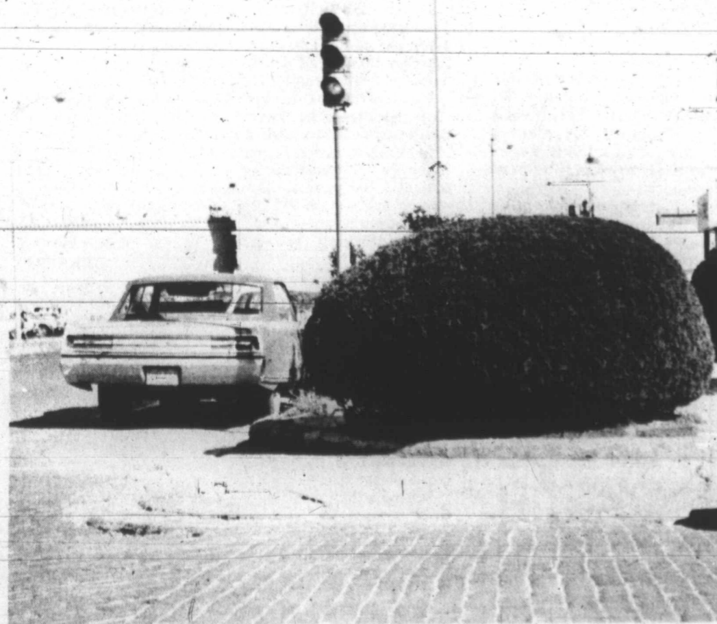
BLIND CORNER — This intersection at the corner of Francis and Frost Sts. is one of the traffic hazards receiving consideration by the City of Pampa in an effort to eliminate driving hazards at "blind corners" throughout the city. The city has reported negligible response from the public in voluntary cooperation for removing the hazards.
