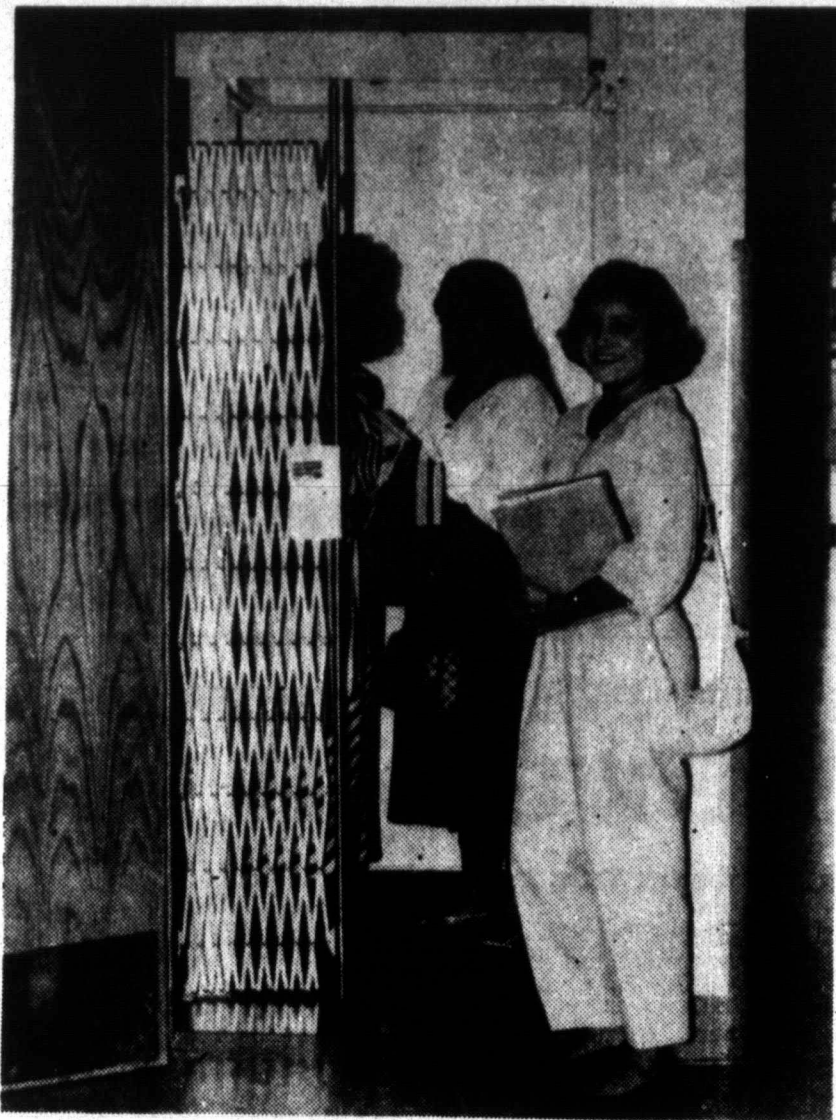
GOING UP? — These three Pampa High School students check out the new elevator at the high school but, alas, they can't use it. The elevator was installed during the summer for use by handicapped students. Left to right are Shannon Churchman, Kelly Finkenbinder and Dusti Fritz. (Staff photo by Deborah Hendrick)
