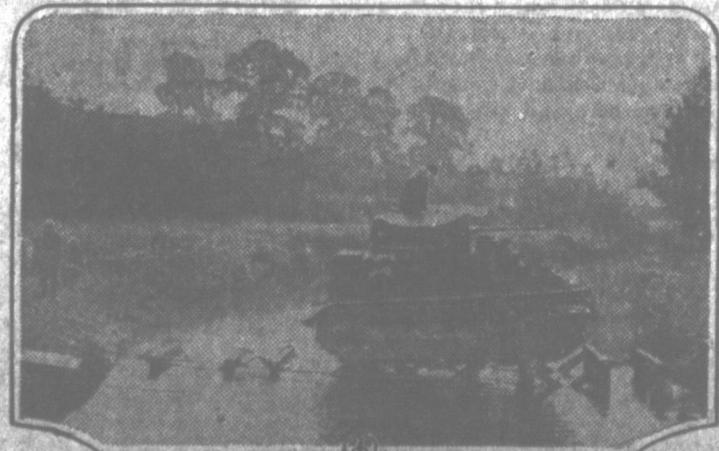
British engineers have found a way for tanks to step across unbridged rivers—by means of specially constructed wooden "stepping stones." Here one of the heavies is shown picking its way across the River Avon, near Amesbury, England.
